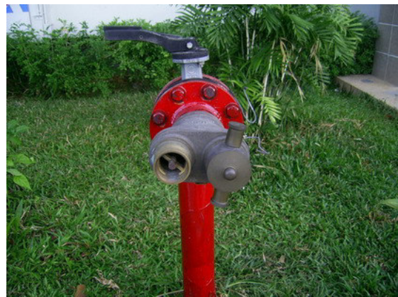
Junk in the drain and found that fire host connection cover lost
