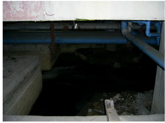
Waste pipe leaked under the building
