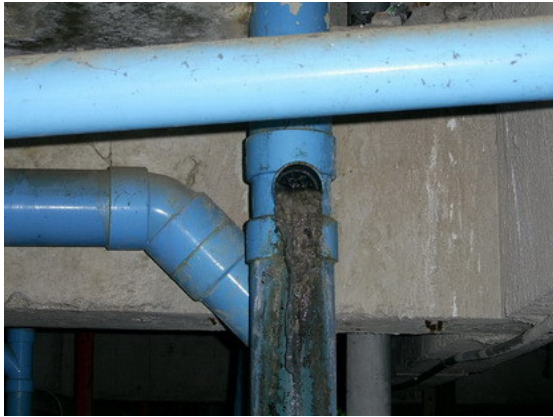
Waste pipe leaked under the building
