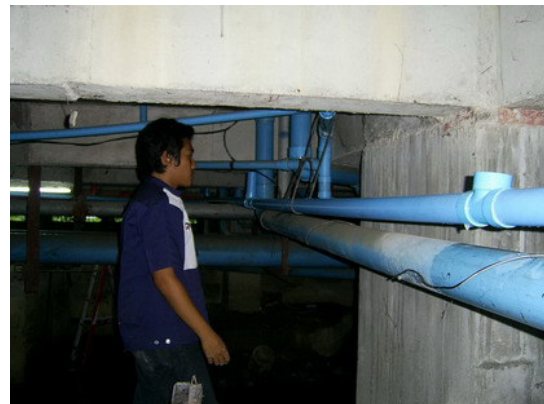
By pass leaking point, no more waste water
