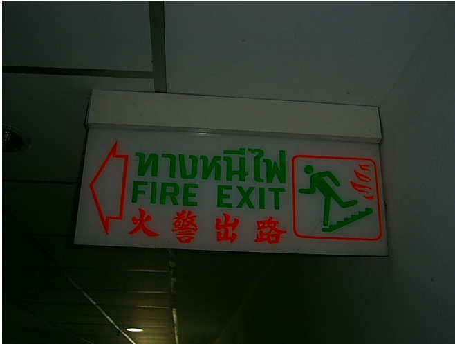
Fire Exit sign
